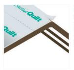
**6.1** Roll out the BreatherQuilt and fix in place using staples. Cut along the centre of the ridge beam and staple to the ridge beam to secure.
