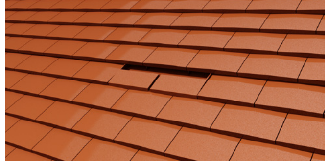
HD TV10/9 Installed
