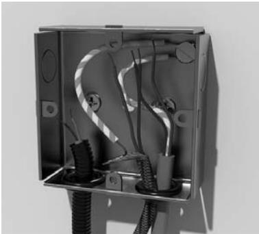
The earth from the mat can then be connected to the earth from the incoming supply by using the earth terminal in the back box. If using a plastic box with no terminal then a terminal block can be used.
