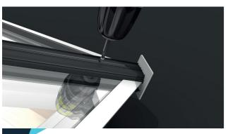
It is important to fit the **longest** pressure plates opposite each other first and screw down into the rafters through the pre-drilled holes in the pressure plates using 4.2mm x 45mm screws.
