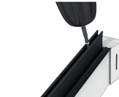
**9** Re-tighten the screw on the top of the hip rafter making sure the joint is tight.
