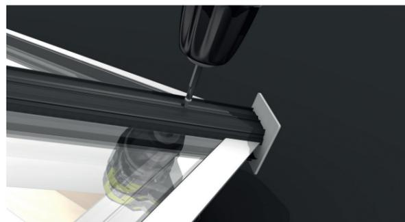
**17** It is important to fit the **longest** pressure plates opposite each other first and screw down into the rafters through the pre-drilled holes in the pressure plates using 4.2mm x 45mm screws.
