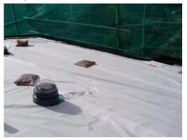
Place protection fleece roll onto roof and lay over waterproof layer in strips from one side of the roof to the other, all the way to perimeter. Start roll again next to previous length of fleece but overlap by 100mm.
