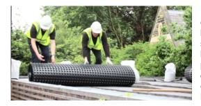
Roll out the drainage board onto roof ensuring a continuous drainage layer is created. Cut drainage board at perimeters of roof leaving a neat edge. If river stone edging is being used at edge, leave a 300mm border between drainage layer and perimeter. Where protruding skylights etc. come through the roof, cut the drainage board up to it and cut around to form neat edge. Be careful to NOT damage the water proofing layer.
