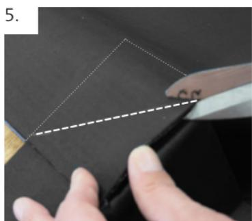
Apply the second flashing strip and make a mitre cut on the upstand parapet.
