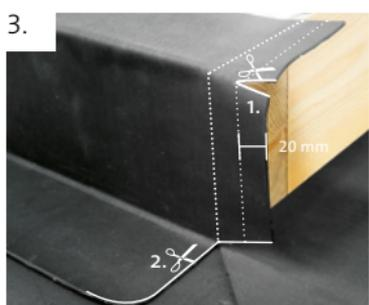
Cut 20 mm into the top projection (1.) and cut into the bottom projection as far as the corner (2.). Form an inverted pleat.
