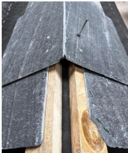
Installation with standard top battens
