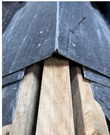
Installation with Ridge runner batten
