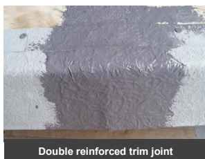
Double reinforced trim joint
