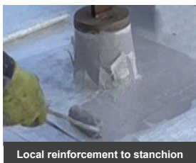
Local reinforcement to stanchion
