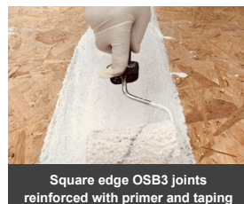
Double reinforced trim joint
