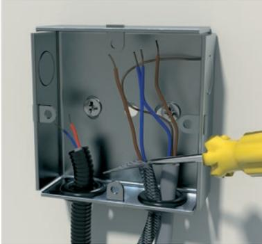
Depending on the type of mat supplied, the cold tail (black lead) may have either a solid earth cable or an earth braid wrapped around the internal cores, this needs to be unbraided by using a screwdriver and pulling down the braid to separate the strands. These can then be twisted into a single strand.
