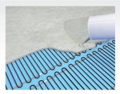
we recommend a minimum of 8mm suitable latex levelling compound to cover the heating mat/cables to ensure even heat distribution.
