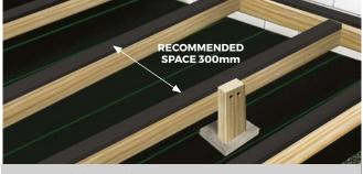
300mm joist spacings are recommended, you should never exceed 400mm spacings.
