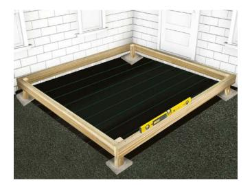
J If your deck will be sitting on grass or soil, you will need to place blocks or slabs underneath each leg, to spread the load and provide a level, stable base. Additional blocks can be used if required. Position and adjust the blocks/slabs, ensuring the frame is at a slight angle, that will allow the water to drain down the length. We recommend a slope of at least 5mm for every metre. Alternatively, if using slabs, you could dig a hole and set the legs in concrete.
