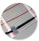
The end joint can be secured in place by taping the red heating element just before the joint to help secure it in place. This will ensure the joint is NOT covered with tape. Both these heating joints MUST now be fully encapsulated within levelling compound and/or tile adhesive.
