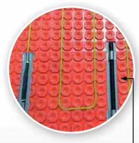
The cold tail joint can be secured in place by taping the cable either side of the joint, a small piece on the heating cable and a small piece on the cold tail. This will ensure the joint is NOT covered with tape.
