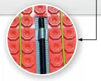
Position the floor sensor in the black conduit supplied between two runs of cable and tape into position. The sensor wire can be shortened or lengthened. If you need to cut the sensor wire you must only cut the end containing the wires. DO NOT cut the end which contains the plastic sensor.
