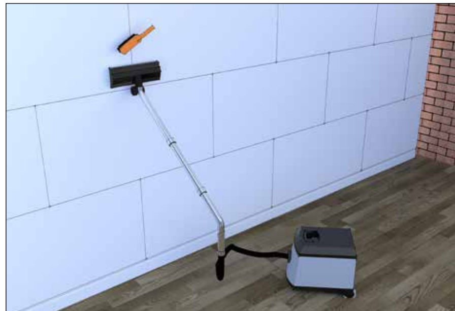
Fig. 7 Preparing Spacetherm WL surface for jointing
