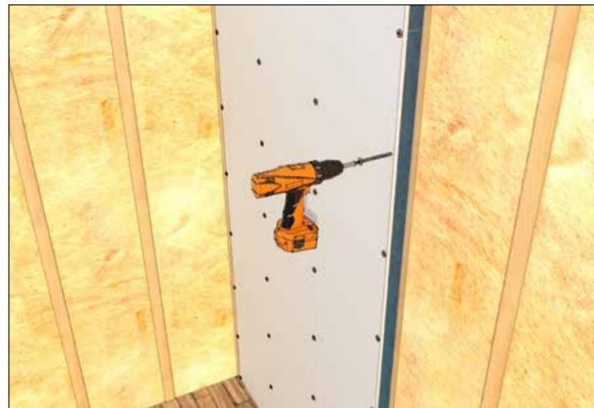
Fig. 4 Fixing Spacetherm Multi to timber straps
