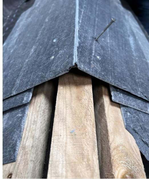
Installation with Ridge runner batten
