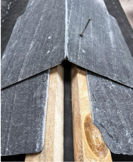
Installation with standard top battens
