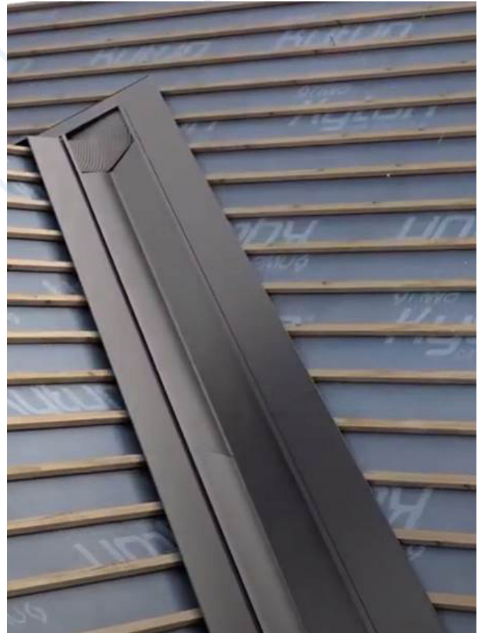
Fig 3. Valley Trough and Trim installed
