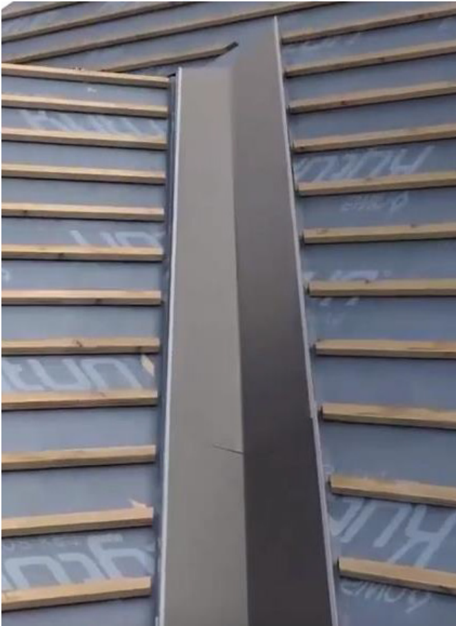
Fig 2. Valley Trough installed
