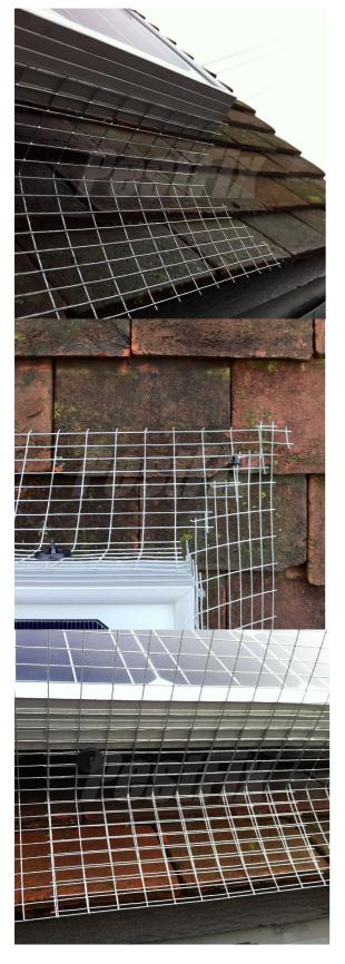
6. Always install the mesh panels starting from an outside corner into the middle of the panel array. Start at each end and work your way towards the middle. Cut the mesh at 45° across the bent section of the panel to form a neat corner.
