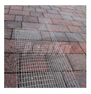
2. Cut the welded mesh roll into manageable section of approximately 2 meters, on the ground. This will make working with the mesh at height easier. Wear protective gloves when handling and cutting the mesh, it will have very sharp edges.
