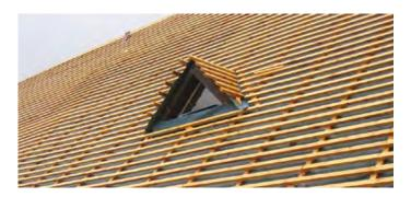
UV Roof offers exceptional UV resistance and is designed for use in partially open roof designs. It is also suitable for shallow pitched roofs with a pitch greater than 5 degrees.
