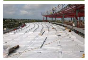
AVCLs act as barriers to prevent moisture within the building's warm air from reaching the insulation layer and forming interstitial condensation. In roof installations, impermeable AVCLs increase the building's air tightness and aid the control of condensation within a roof space.
