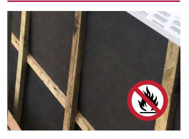
Flameout Breathe membranes are engineered with superior flame retardant properties. Flameout Breathe Class A is the only Euroclass A (non-combustible) breather membrane in the UK.
