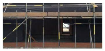
Powerlon SupaPerm SP100 is a single layer non-woven fabric that is both breathable and water resistant to BS 4016.
