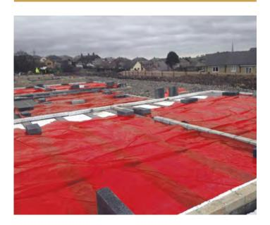
Powerbase is a range of geosynthetic barrier membranes for protection against hazardous gases in covered installations. They are also suitable for groundwater and environmental protection installations.
