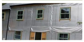
Powerlon ThermaPerm breather membrane has a thermo-reflective layer for improved energy performance.
