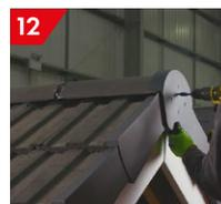
12 To finish, twice screw fix the Ridge End Cap to the ridge batten, securing it in place and completing the Ambi Dry Verge system. The ridge system will need to be installed prior to fixing this. If required a small slot can easily be made on each side of the end cap so it sits over the upstand of the verge unit.
