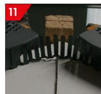
11 Insert Ridge Closer into the last unit - When we reach the top or apex of the roof, we can close this area off by using the ridge comb that is supplied as part of the eave and ridge kit. The teeth of the comb sit over the bottom edge of the verge unit where it will be held in place. If using a dry ridge system the ridge roll can be extended over, tucked back up and stuck to the underside to offer additional protection.
