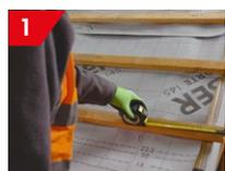
1 Extend the tiling batten -Once the roof has been felted, you will need to install the tiling battens, ensuring they are extended 35mm beyond the gable wall, barge board or render. This will allow for screw fixing the verge.
