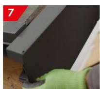
7 Fit the first verge section making sure that it is located firmly onto the eaves starter.
