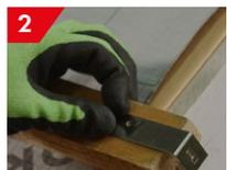
2 Alternatively you can fix the verge units using a ring shank nail. This should be fixed through a Batten End Clip, which should be fitted to the end of every batten, and would require a smaller overhang of 25mm.
