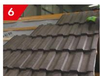
6 The roof is now ready for tiling in the normal way, ensuring the tiles finish flush with the end of the batten.
