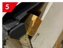
5 An additional batten behind the fascia board can also be used if required to ensure a suitable fixing point - this should be securely fixed to the rafters.
