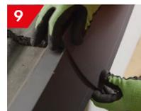
9 The second verge can easily be positioned by locating the front edge of the verge over the two notches on the installed verge, and sliding up until it meets the leading edge of the tile.
