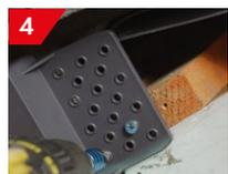
4 The eaves starter unit should be twice fixed to the end of the fascia board, brickwork or timber tilt fillet.
