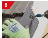
8 Once in position the verge unit can be screw fixed into the end of the batten using flat headed screws.
