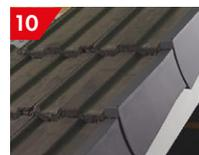
10 This process can now be repeated, ensuring each verge unit engages with the one below, so a verge unit covers the end of every course of tiles.
