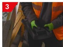
3 Fix the eaves closure -Next, you will need to fix the Eaves starter. Establish the position of the starter unit by making a mark by positioning it inside a verge unit and placing it in position, flat on top of the tile. Now remove the eaves starter prior to fixing.
