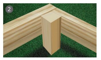
To raise the frame, cut four blocks of 100 x 100 green treated timber to the desired height. Screw these to the inside of the frame at each corner, ensuring they're flush with the top. These legs will be taking all the weight for now so ensure they are properly secured to the frame
