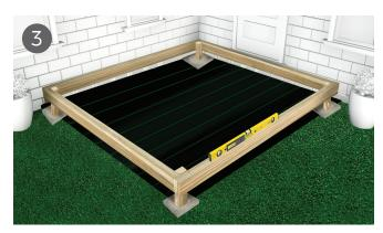
If your deck will be sitting on grass or soil, you'll need to place blocks or slabs underneath each leg to spread the load and provide a level, stable base. Position and adjust the blocks/slabs, ensuring the frame is at a slight angle that will allow the water to drain down the length. We recommend a slope of at least 1 in 80 (1cm drop for every 80cm of distance). Alternatively to using slabs you can dig a hole and set the legs in concrete.
