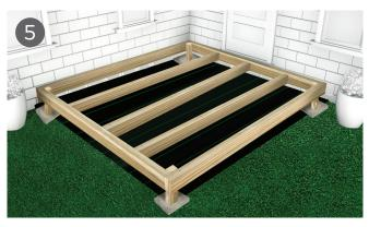
Measure across the inside of the frame at your joist marks, then cut lengths of the green treated (47mm x 100mm or 47mm x 150mm) timber to suit. To fix the joists, tap them in with a hammer until flush with the top, ensuring they do not push the frame out of shape, then screw them in place from the outside of the frame.
