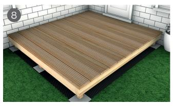
Lay the second board next to the first board and continue this pattern of laying until you reach the end of the frame area. If your project is on a curve or slight angle, you may need to use a circular saw to finish off any overhanging edges. If you're adding Fascia boards, you must allow for a slight decking overhang. When fixing the timber decking, pre drill all boards with a 2mm bit, to prevent boards from splitting. For a smooth finish counter sink all fixings.
