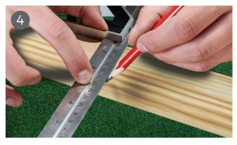
Mark across one side of the frame first every 400mm, this will set you joists at the maximum required 400mm centres then repeat the process on the opposite side of the frame. You may wish to set your joists at smaller than 400mm centres to ensure even spacing of the joists across the frame.
