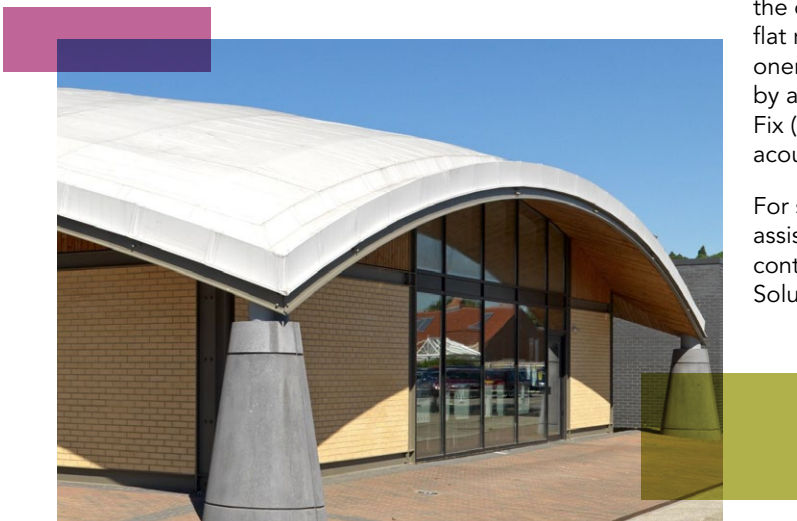
Image courtesy of GSS Architecture - www.gssarchitecture.com
