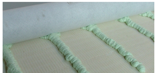
A bonded membrane incorporating HardRock Multi-Fix (DD)
