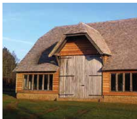
Hardrow® Slates Duets® Barley on a Barn Conversion at Chesterton, Oxon
