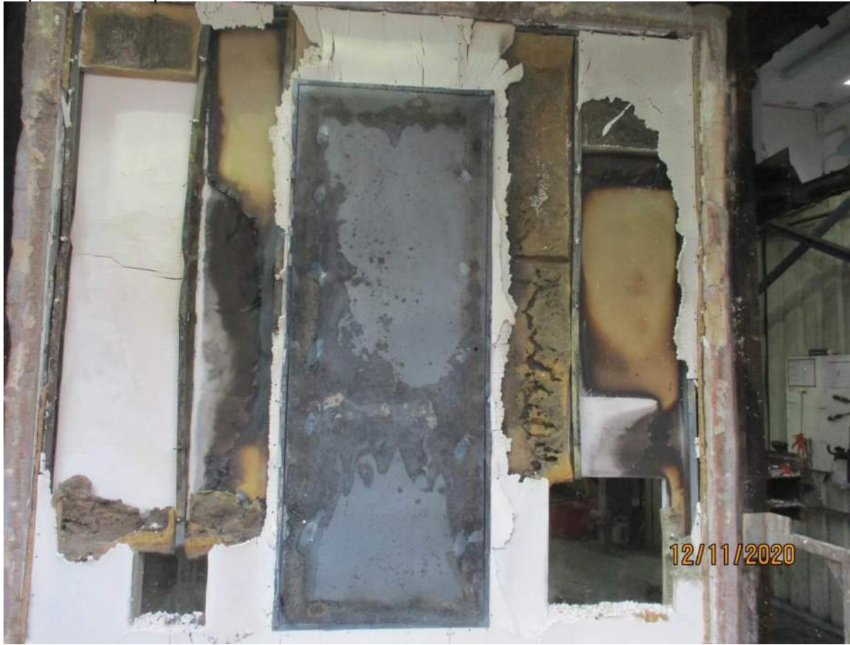
Exposed face – post test
