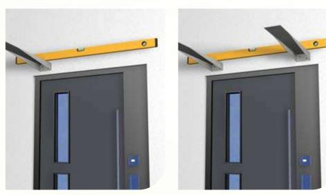
**3.** Level the wall bracket with a spirit level and check the position of the second wall bracket. Fit the second bracket into position. Double-check level after fixing, and adjust or pack as required.
