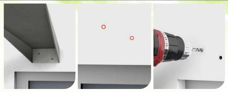
1. Position canopy and mark the wall bracket location. Using the two holes provided mark the fixing holes with a pencil or permanent marker. Drill holes to suit the chosen fixing method, anchor bolts or chemical anchor fixing is recommended.
