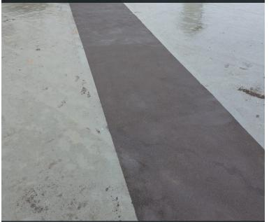
100lm of walkways installed over the completed Fastcoat Pro roof using LRS Fastcoat Pro Traffic Coat
