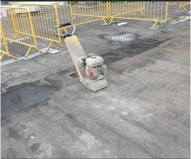
Scabbler used to remove the stone chippings that were embedded into the surface
