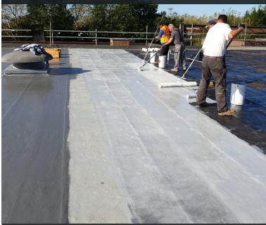
Base Coat and Reinforcement Matting being embeded into the base coat of FastCoat Pro
