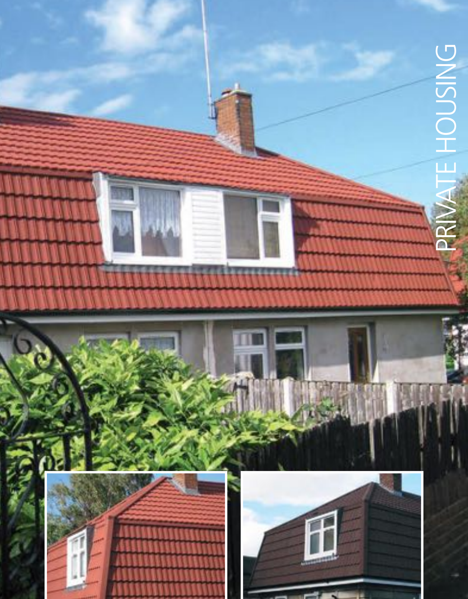
Complex ridge detailing using Metrotile barges & end cap accessories
