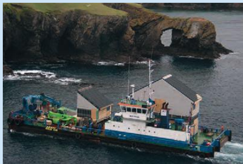
Top: Work continues assembling the pre-constructed pods Centre: The site as seen looking towards the sea Bottom: Pods arriving by sea aboard the MCS Ailsa
