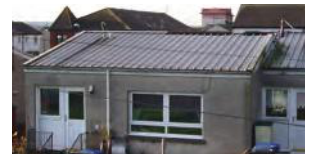
Roofing prior to refurbishment
