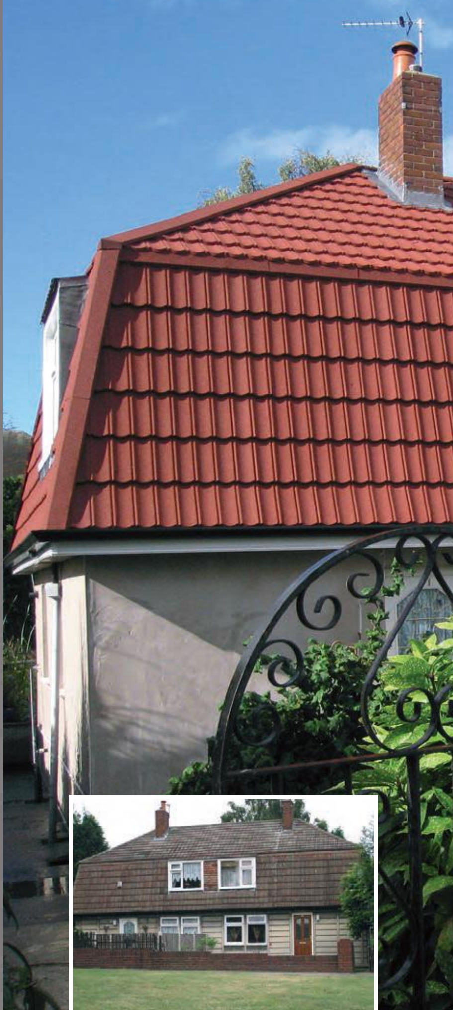
Old roofs before installation
