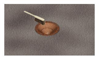
**Step 1**Remove redundant roofing materials; brush & clean surfaces ready for new installation.
