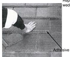
Repositioned slate Slate wedge wedge SLATE 2
